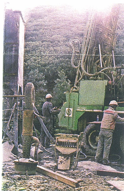
Drilling the Iron Mountain Mine
